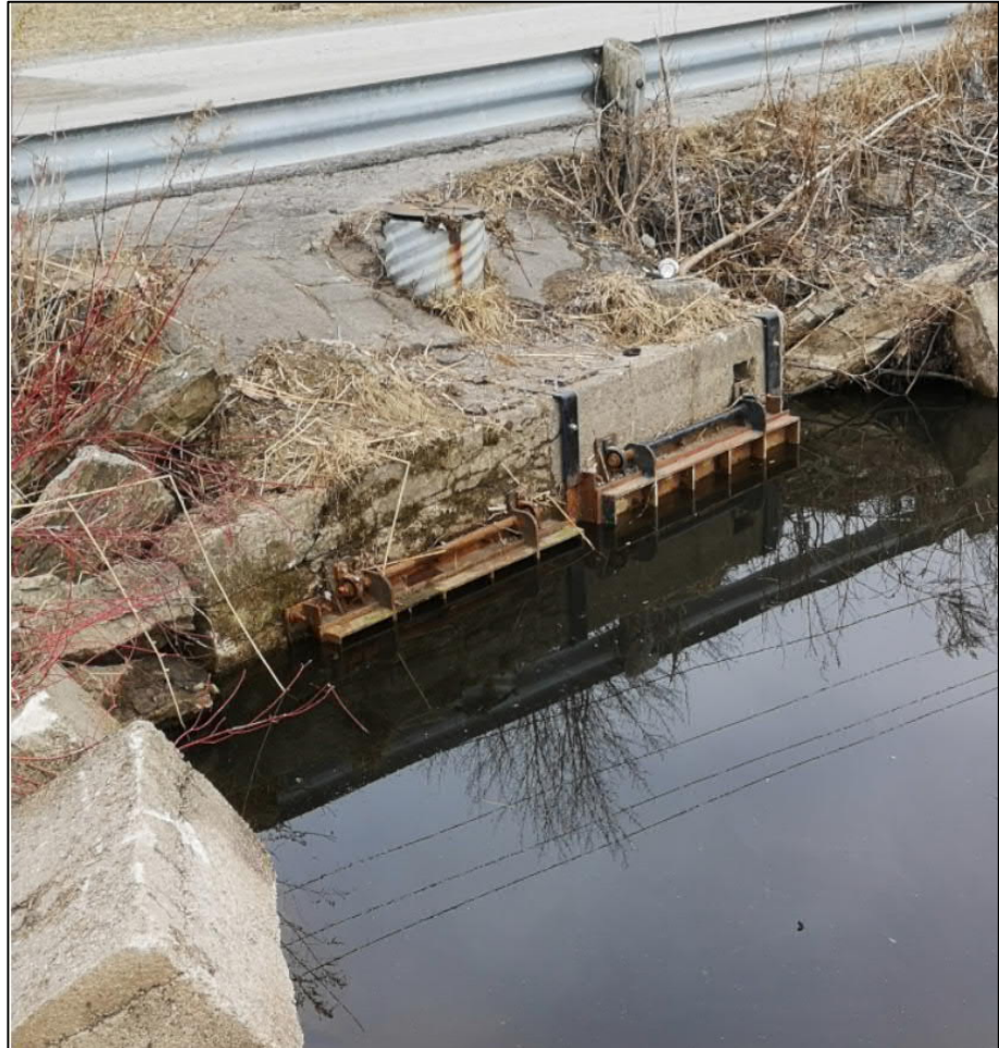
Figure 27 Point Abino Drain Outlet
