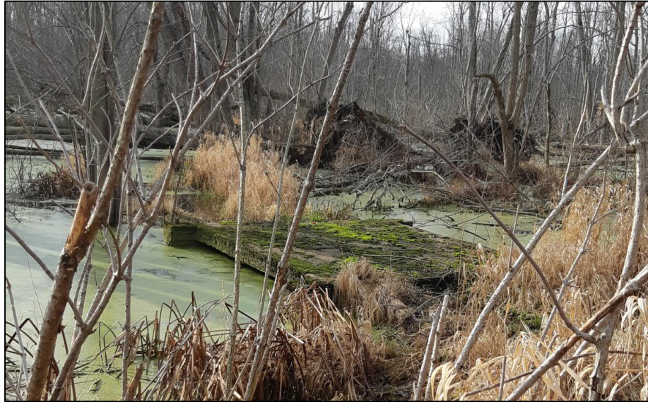
Figure 33 Mathews Rd S Drain Crossing PAM-CS-03
