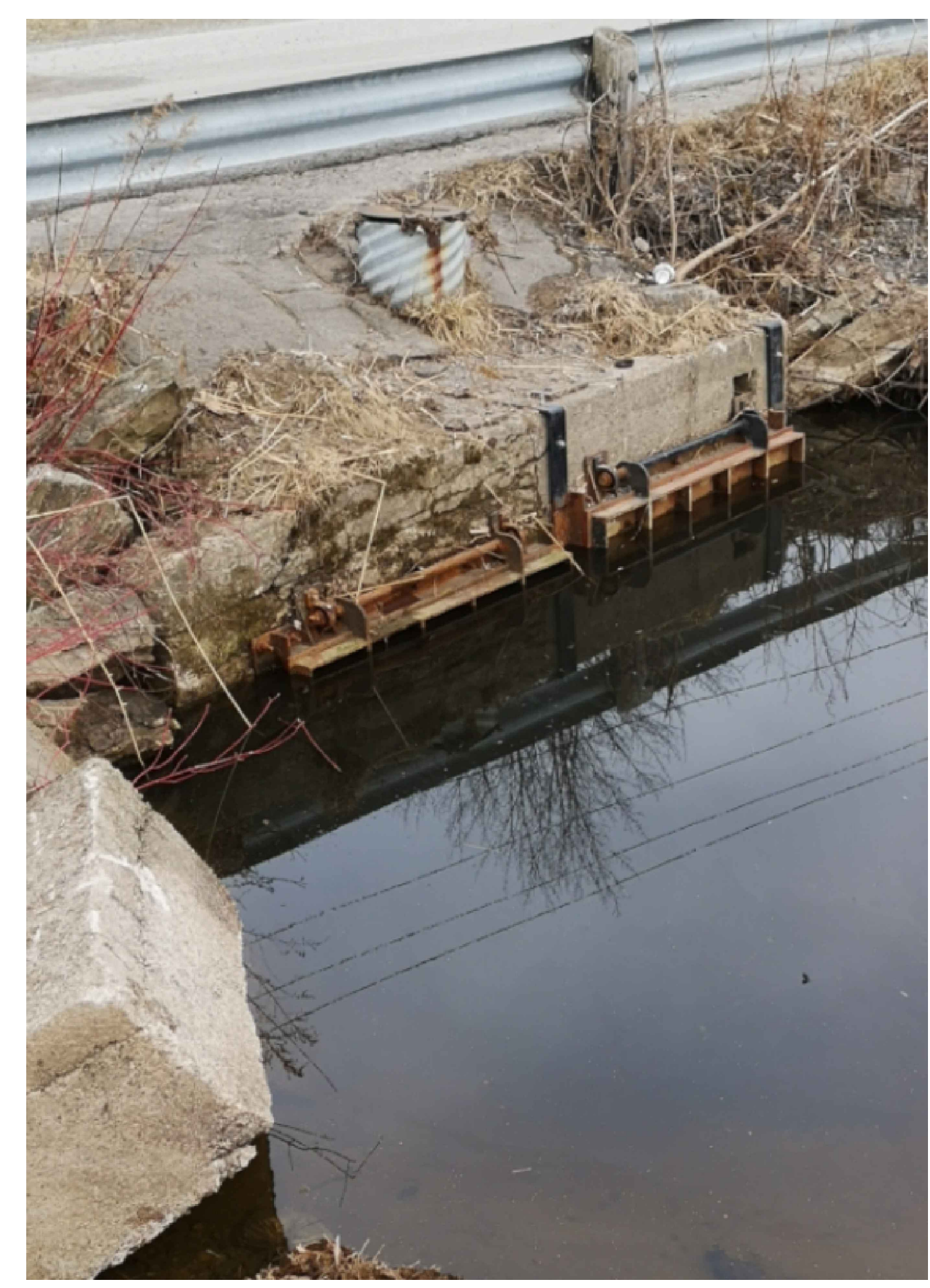
OUTLET OF CULVERT
