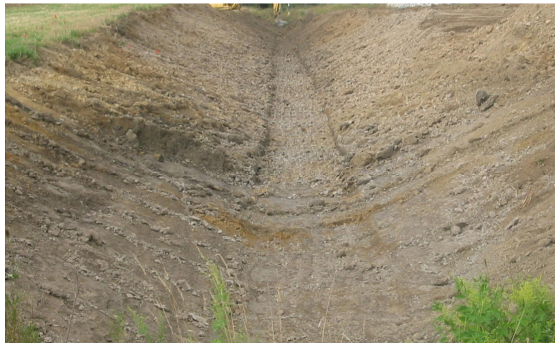
Figure 6 Trapezoidal Ditching Under Construction
